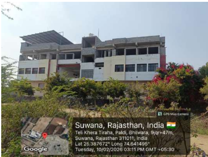
College Building Rear View
