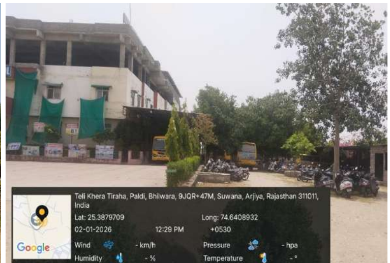
College Building Right View
