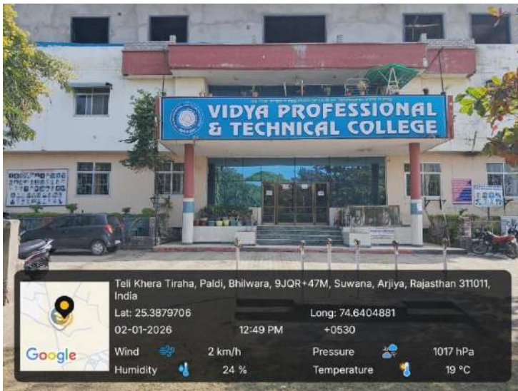
College building Front View
